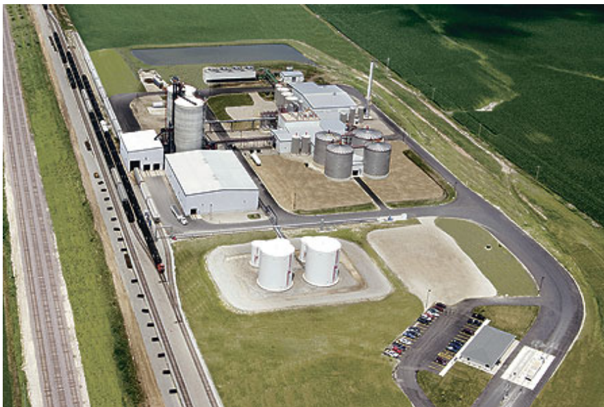
Golden Grain Energy in Mason City, Iowa, is tripling the size of its rail yard to ship ethanol more efficiently.
